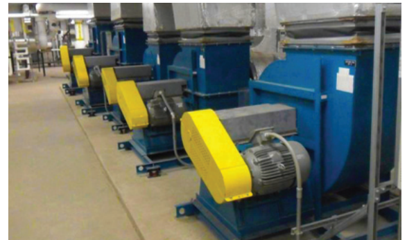
Figure 6: Installed on a VFD-controlled motor in an air handling unit at a community hospital in suburban Chicago, the AEGIS™ SGR Bearing Protection Ring reduced harmful shaft currents by 83% to levels well below those that damage bearings.
