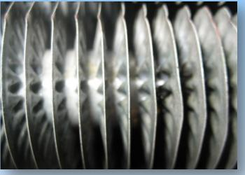
Close-up of coil after conventional cleaning (note: black tar like substance is biofilm) Close-up of coil after proper cleaning
