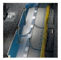
Snake Bus Power Distribution is a prewired, modular power distribution system for access floors. Snake Bus delivers 50 amp, three-phase,
