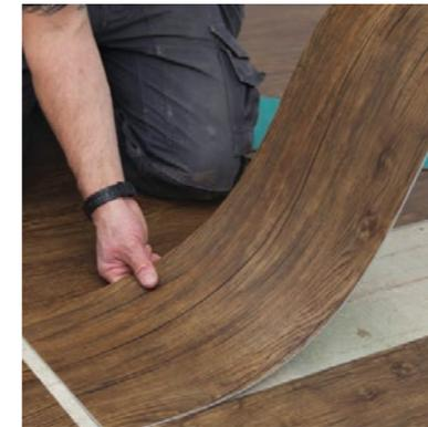
Featuring 59-inch planks, LooseLay Longboard is a non-interlocking floating floor range, notable for its multi-directional planks,
