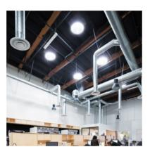
Integrated LED Light Kit allows the integration of natural light and traditional electric lighting from a single fixture for a cleaner ceiling appearance
