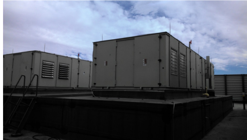
Two of the four existing 75 ton HVAC units
