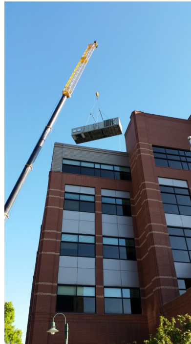
New Unit Going Up!
