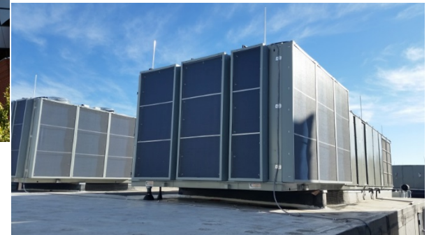
New Units with Evaporcool System
