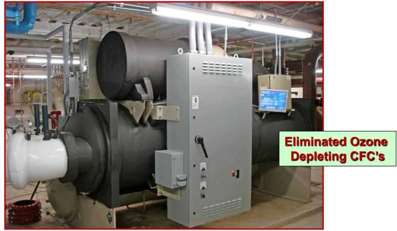
**New 750 Ton High Efficiency Chillers** 2 Chillers – 975,000 kWh Annual Energy Reduction
