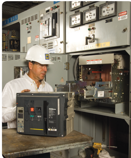
Aging or obsolete circuit breakers (left) are replaced with state-of-the-art circuit breakers, which brings the existing line-up to current technology (right).
