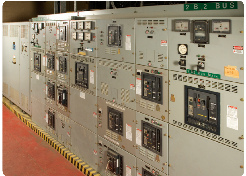
The switchgear structure, conduits, cabling and footprint are left intact, which saves time and money (above).
