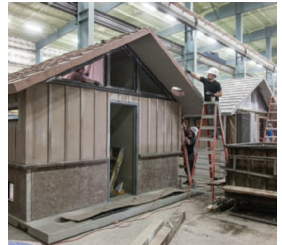
Ending the condensation problem saved time formerly spent protecting product finishes.
