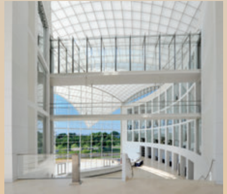
Integrated systems help meet the climate-control challenges of an enormous atrium.
