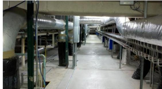
**Figure 3: Straight duct and pipe runs within interstitial space**
