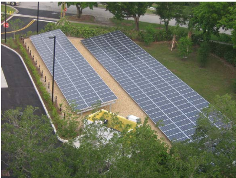
Net Zero Energy Store Ground Mounted PV Field Ft Lauderdale, FL
